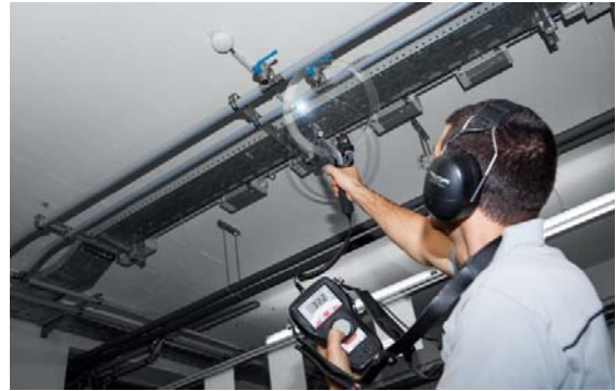
Figure 9: Detection of leakages in the distribution of compressed air
